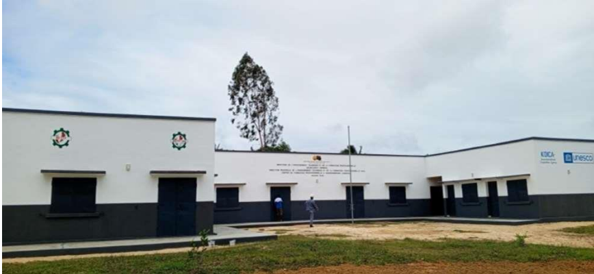
The Vocational Training Centre located in the city of Sambava, comprising 6 training rooms, 3 offices for administrative staff and 2 practical work rooms furnished and equipped by UNESCO © UNESCO
